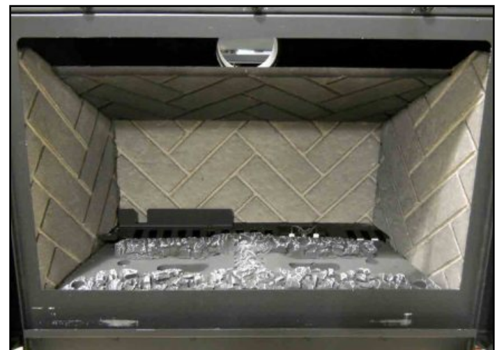
Figure 10.8 Refractory Installed
