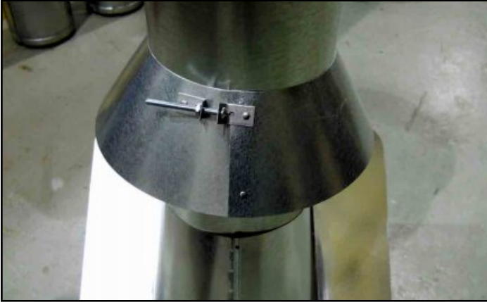
Figure 7.14 insert Bolt into Brackets
