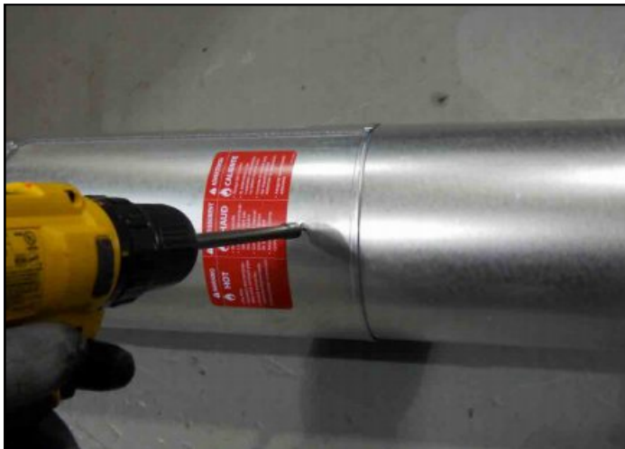
Figure 7.4 Screws into Slip Section
