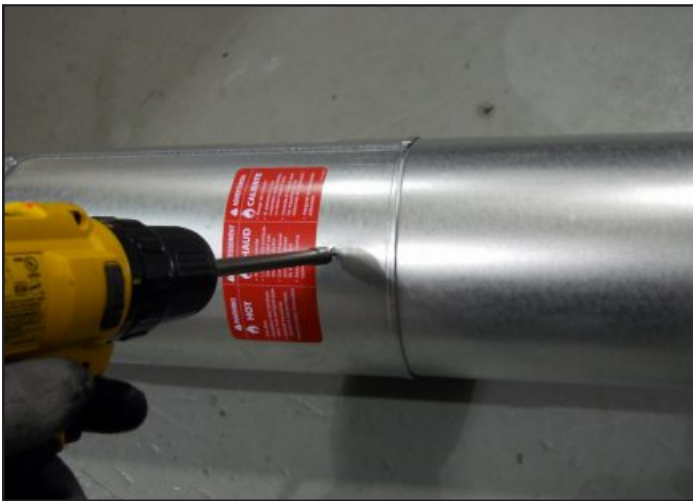
Figure 7.4 - Screws into Slip Section
