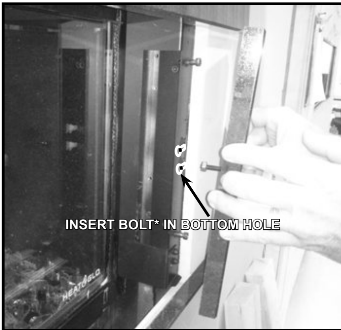
Figure 10.25. Install Side Granite Pieces
