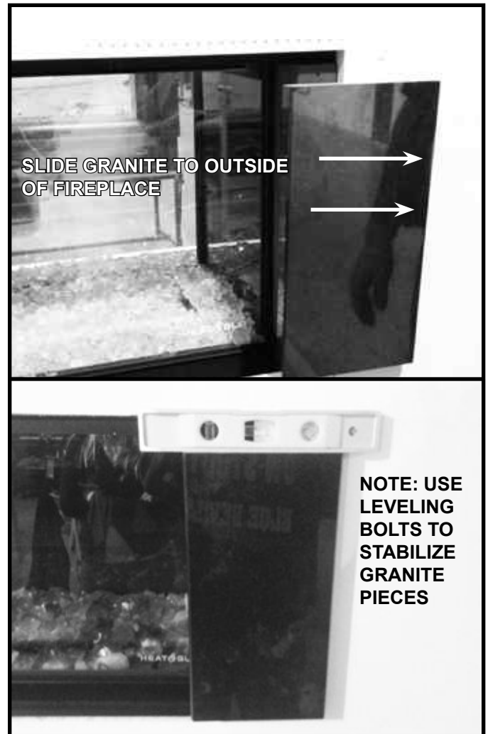
Figure 10.26. Right Side Granite Piece Installed and Levelled
