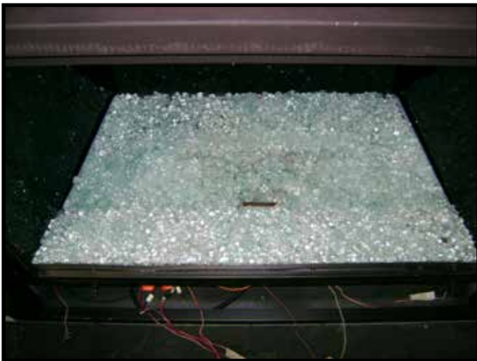
Figure 14.9 Proper Placement of Media
