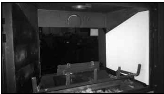
Figure 2. Install Rear Glass Panel
