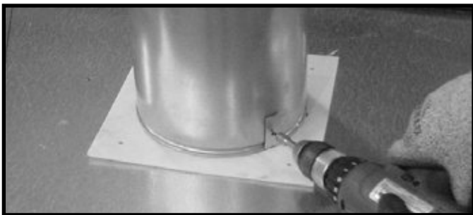
Figure 6.6 (Generic Fireplace Shown) To attach the first section of vent pipe, make sure to use the fiberglass gasket in the manual bag to seal between the first vent component and the outer fireplace wrap. Caulk with a minimum of 300 °F continuous exposure rating may be used to hold the part in place.
