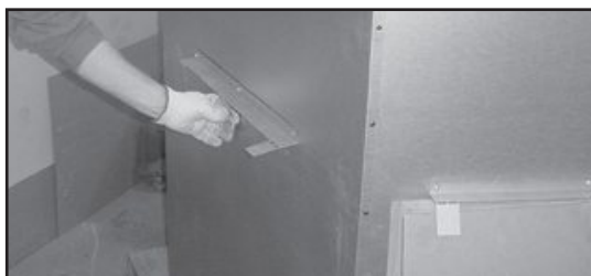
Figure 3.7 Bending Refractory Shipping Tabs Back Down
