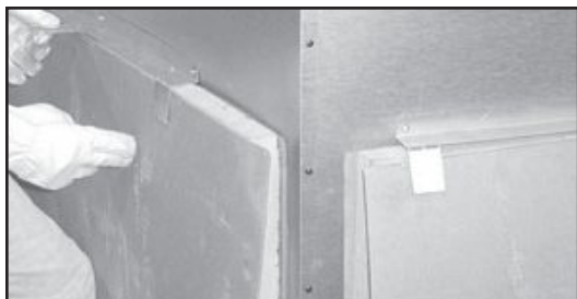
Figure 3.6 Unpacking Back Refractory
