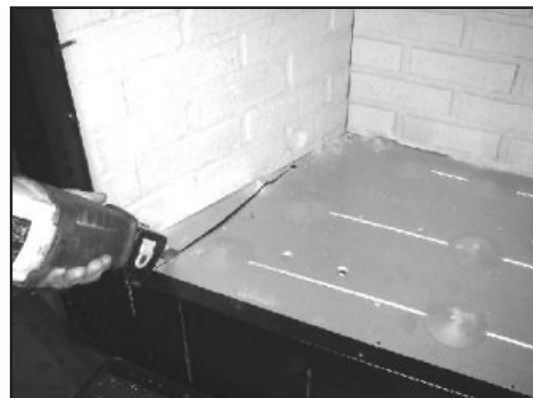
Figure 12.3. Using a saws-all, cut out the floor.
