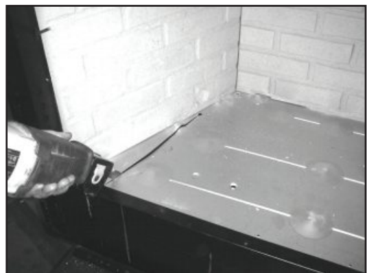
Figure 10.3. Using a saws-all, cut out the floor.
