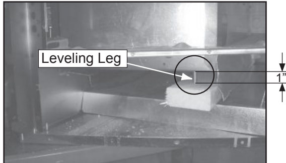
Figure 11.2. Ensure that the leveling leg is positioned over the 2 x 4 before leveling the insert. Minimum 1” clearance.
