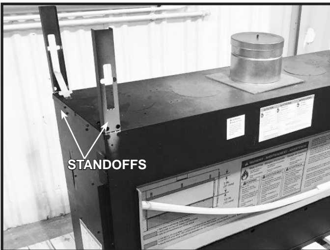
Figure 6.2 Standoffs in Vertical Position
