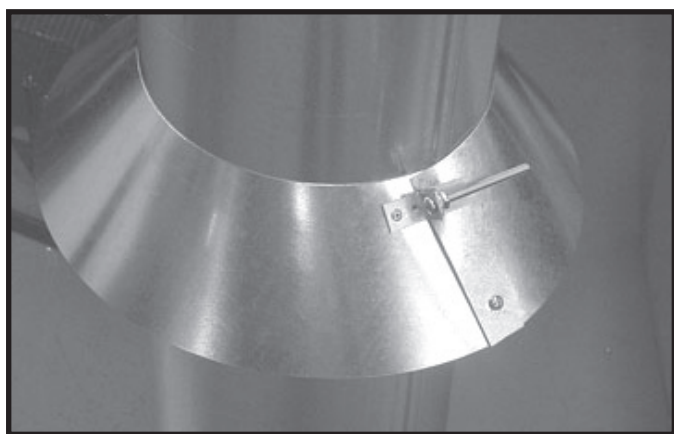
Figure 7.13 insert Bolt into Brackets
